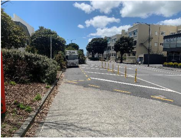
Figure 2-57: Embankment down to road
