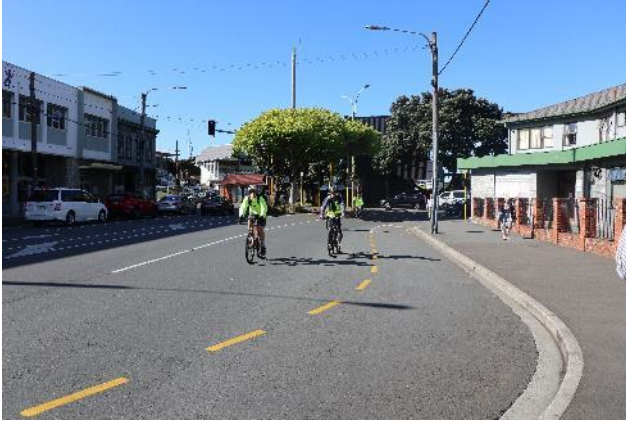
Figure 2-25: Typical cycle use observed (southbound movement)
