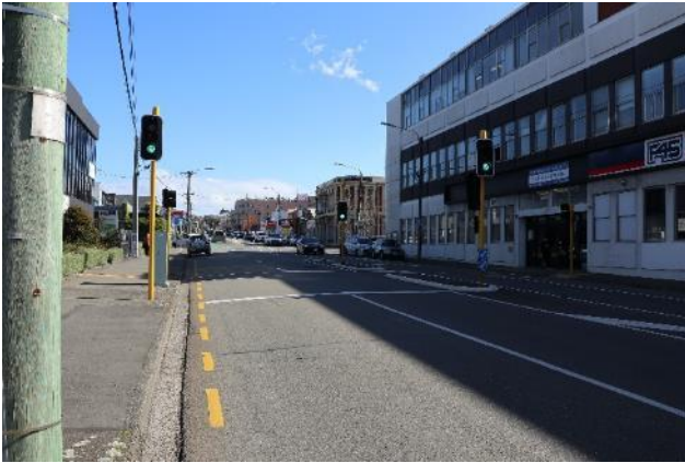
Figure 2-21: Existing mid-block pedestrian crossing. Note access under building.
