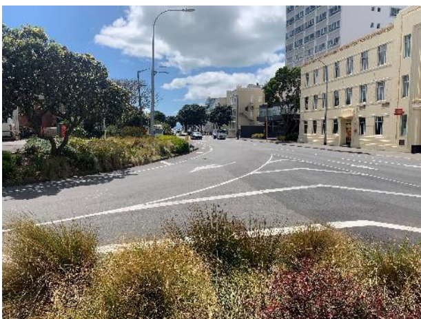
Figure 2-59: FENZ Fire Station right hand side
