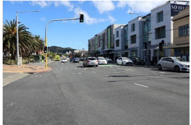
Figure 2-14: Hospital Access: Note limited guidance to motorists of cycle movement over the access side road.
