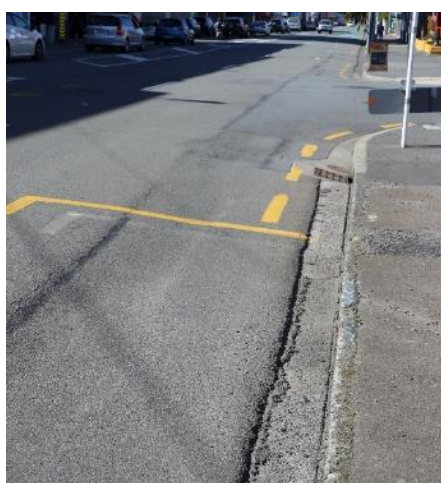
Figure 2-1: Example of rolled lip to seal edge Figure 2-2: Example of rolled lip to seal edge
